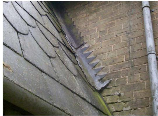
**Photograph 5: Lifted tile and gap under lead flashing**
